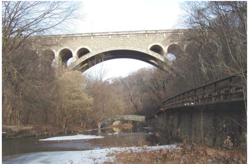
Henry Avenue Bridge over Wissahickon Creek (1927 – 1932)
