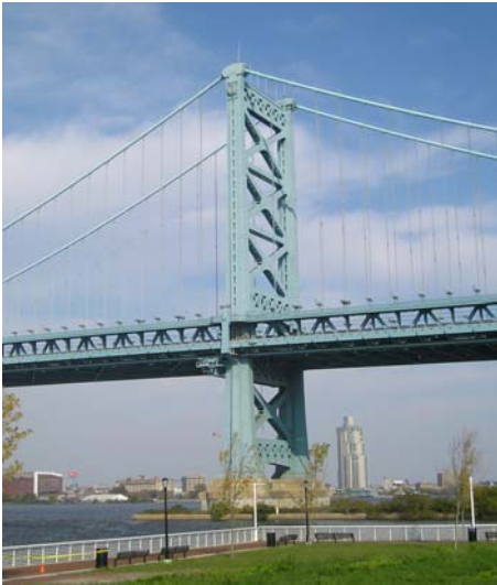
Benjamin Franklin Bridge (1921 – 1929)
